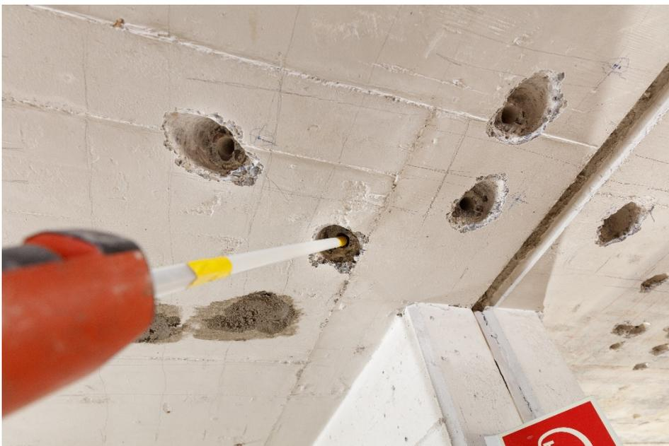
Fig. 27 Injection of mortar (Start position)
