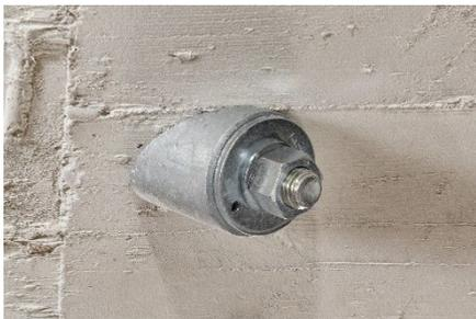
Fig. 9 External anchor head
