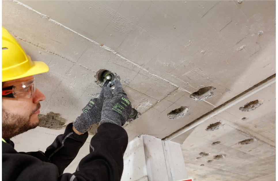
Fig. 30 Installation of anchor head
