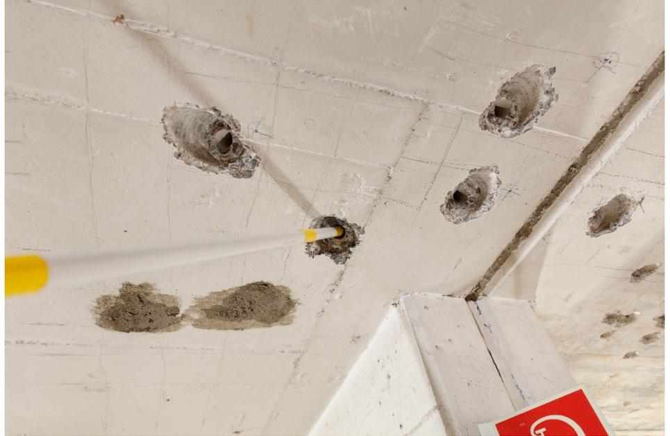
Fig. 28 Injection of mortar (End position)
