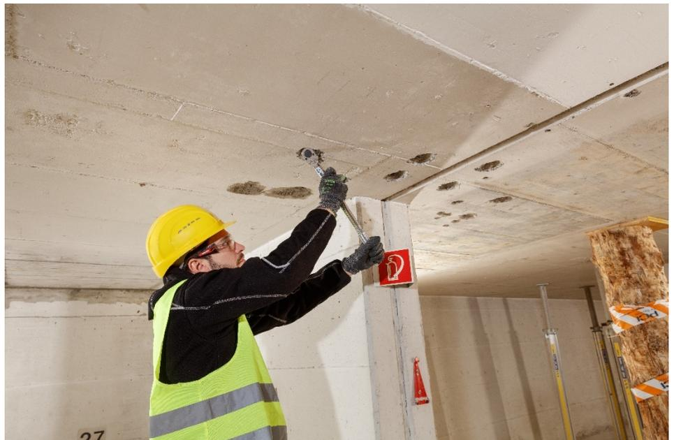
Fig. 31 Application of torque moment
