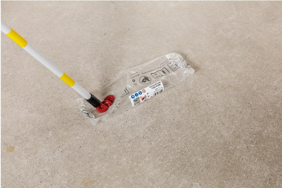
Fig. 26 Discarding of initial amount of mortar
