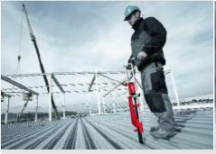
Faster progress: Work quickly and comfortably with the SDT 30 stand-up tool.
